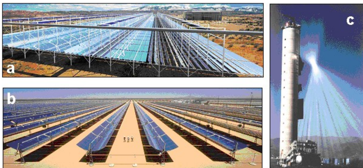
Figure 2: Concentrating solar collectors: a) Fresnel type line concentrators of Solarmundo NV, b) parabolic trough concentrators, c) point concentrators with tower for the receiver volume.
